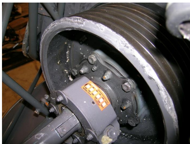
Figure 8: Scratch marks on the upper belt pulley. Photo: AIBN
