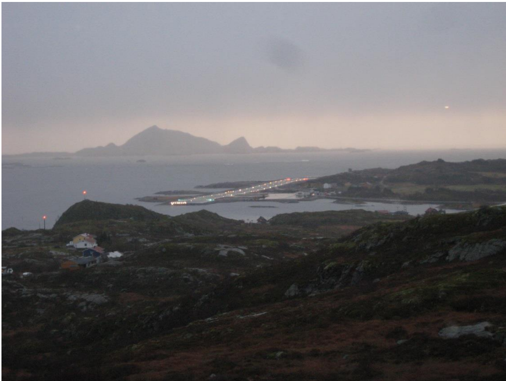
Figure 6: Illustration photo ENSH, seen from the northwest (runway 19). Note red obstruction lights north of the airport. Photo: Avinor
