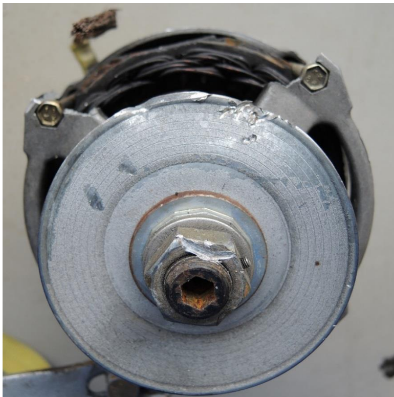
Figure 17: The generator pulley was bent as a result of the impact. The broken generator casing can be seen at the top of the photograph. Photo: AIBN
