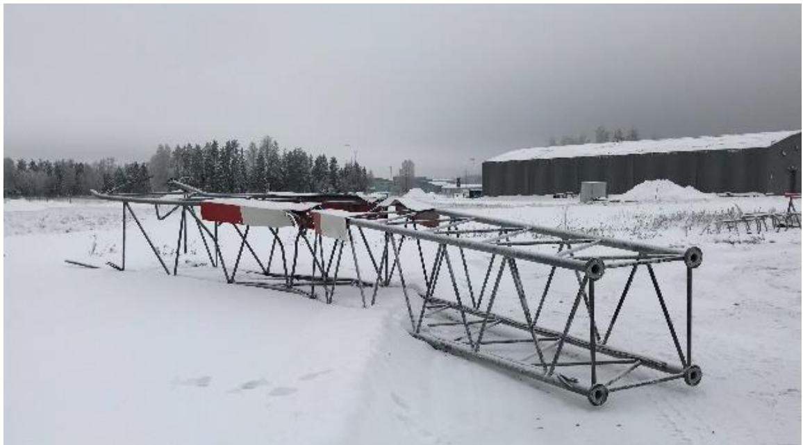
Figure 6: Damage to the light mast (after dismantling). Photo: AIBN
