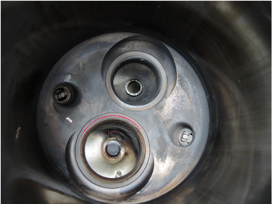
Figure 8: Inside of cylinder no. 5 after the valves had been removed. The undamaged part of the intake valve seat is marked with a red line. The damaged part is darker/brown. Otherwise, it can be noted that the cylinder is clean and has a light color. Photo: NSIA
