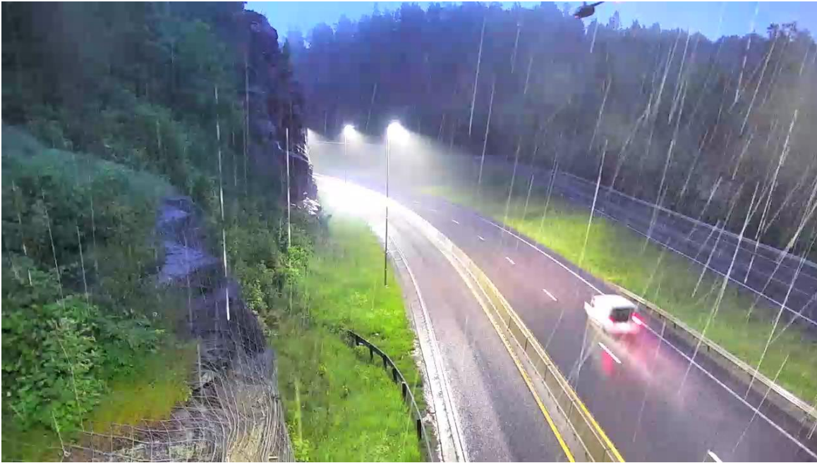
Figure 3: Still image from video. The helicopter appears at the top of the image. The image may give the impression that there was more daylight than what there actually was. Video: NPRA/NSIA
