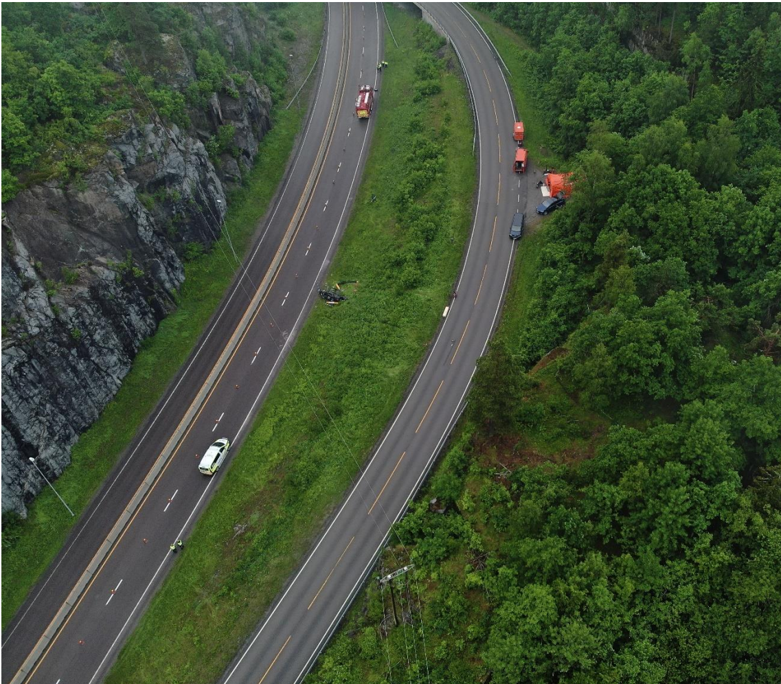
Figure 7: South-easterly view of the accident site. The E18 is the road on the left. The helicopter wreckage can be seen in the centre of the photo. The one remaining conductor and the earth conductor are visible in the photo. Photo: Porsgrunn fire and chimney sweep service/NSIA
