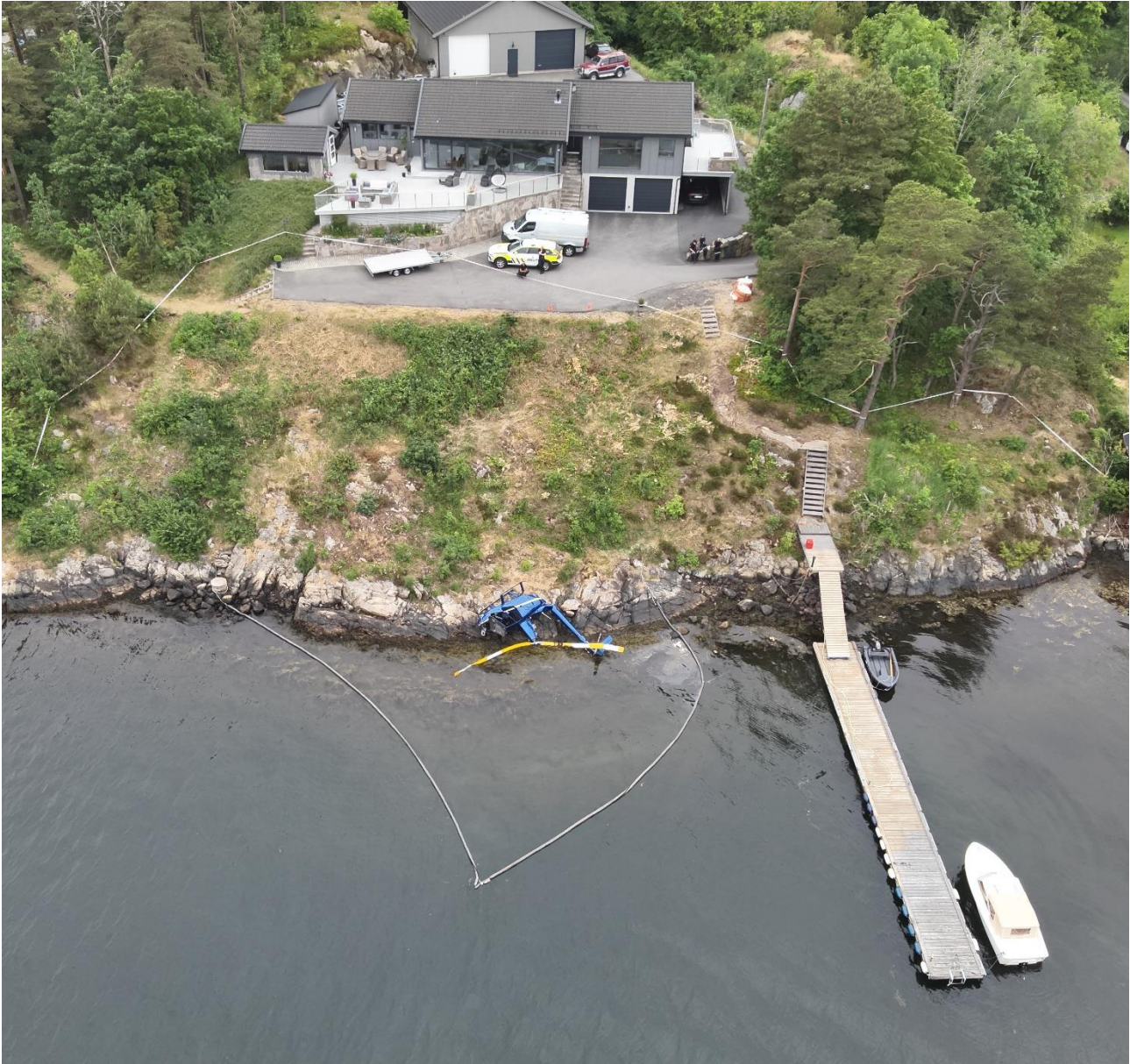
Figure 2: The photo was taken approximately one hour before the full ebb-tide. The two orange cones at the edge of the tarmacked area represent points where the mid-section of the helicopter's skids was in contact with the ground. The two vehicles were not at the site at the time of landing. The witness who filmed the crash was standing on the veranda seen at the top of the photo. Photo: The police / NSIA
