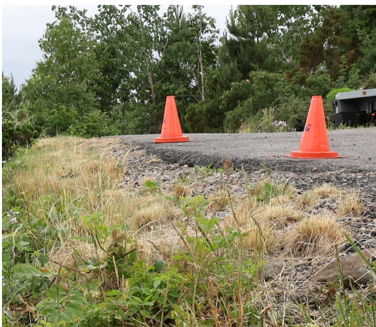
Figure 3: The edge of the tarmacked area where the helicopter landed. See Figure 2 for the location of the cones. Photo: NSIA
