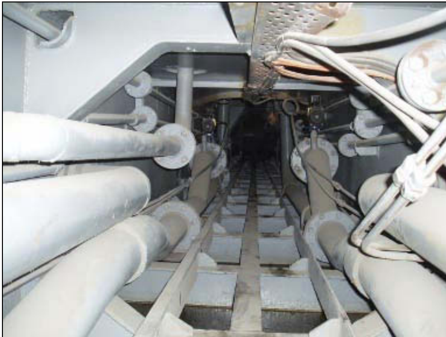
Figure 14: Photo of the pipe trunk.
