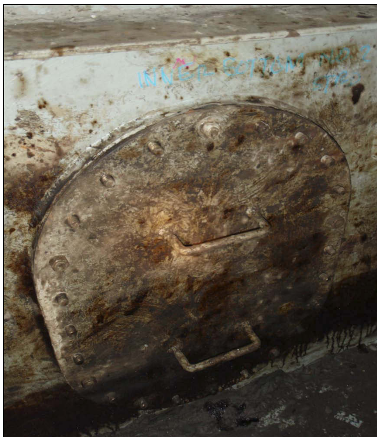
Figure 16: Manhole cover for access to void.
