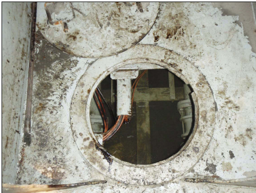
Figure 10: Connection between the blow-tank tunnel and the pipe trunk.
