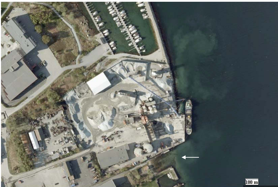
Figure 6: The quay facility at Forus with ship at the quay. The white arrow indicates the area where the deceased was found. Source: Norwegian Coastal Administration
