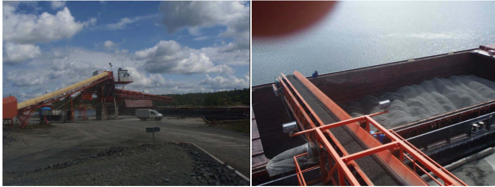
Figure 15: Conveyor belt loading at Stjärnökrossen.
