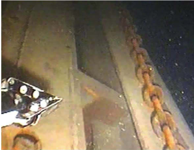
Figure 22: Traverse chains for excavator. Picture from port side. (Photo: KBV)
