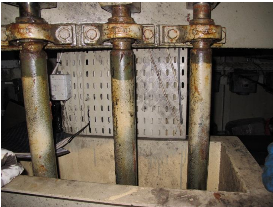
Figure 17: Top of trunk on the bridge deck through which the rods pass through the superstructure down to the engine room. Photo: AIBN
