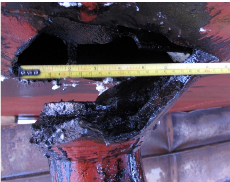
Figure 22: The rear inner strut on the starboard side had torn open the skin of the hull. Photo: AIBN
