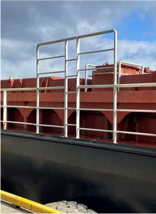
Figure 14: Higher railings installed locally on similar vessel (seen from the quay). Photo: Berge Rederi AS
