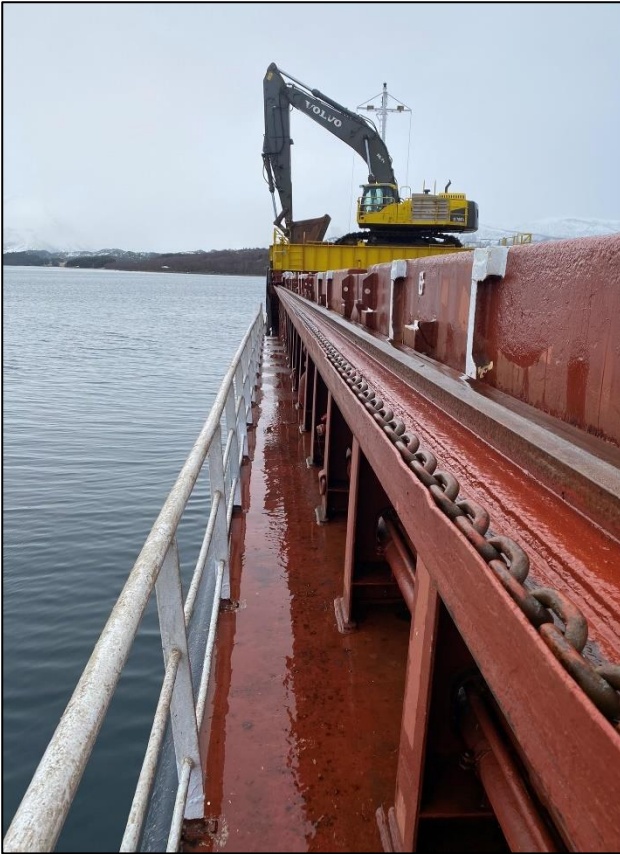
Figure 4: Passageway on the main deck along the cargo hatches. Photo: NSIA
