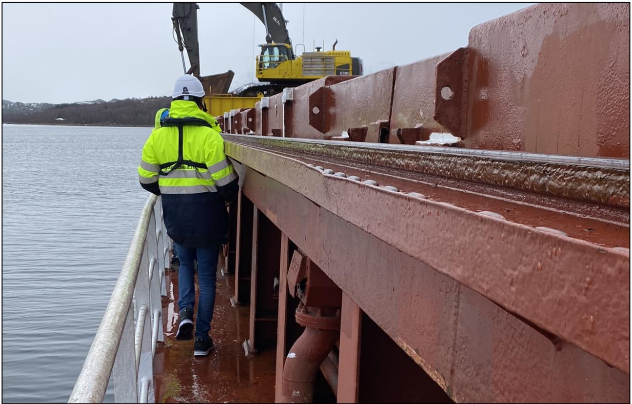
Figure 11: The main deck relative to the hatch deck. Photo: NSIA
