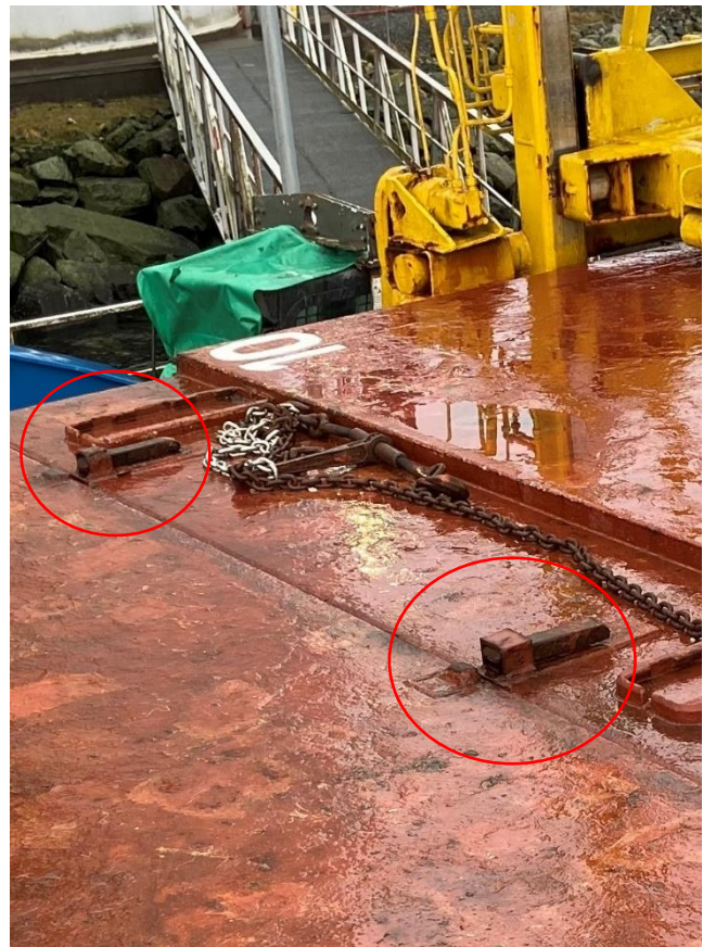
Figure 10: Wedges (see red circle) that ensure that each cargo hatch is fastened to the adjacent hatch. The chain was used to fasten the bucket to the excavator. Photo: NSIA
