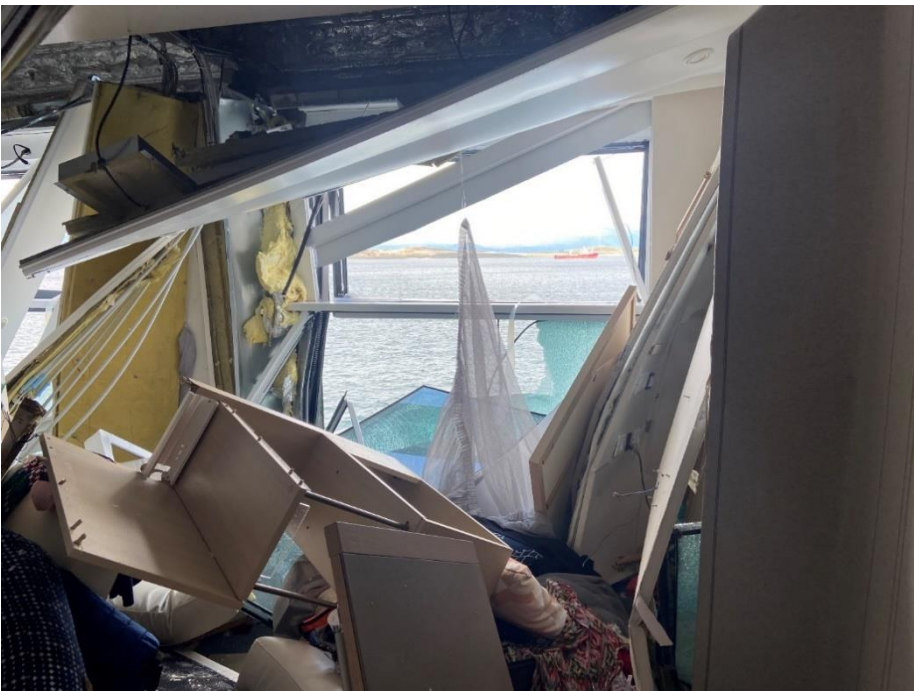
Figure 23: Damage to window, frame and stateroom 2012. Photo: NSIA
