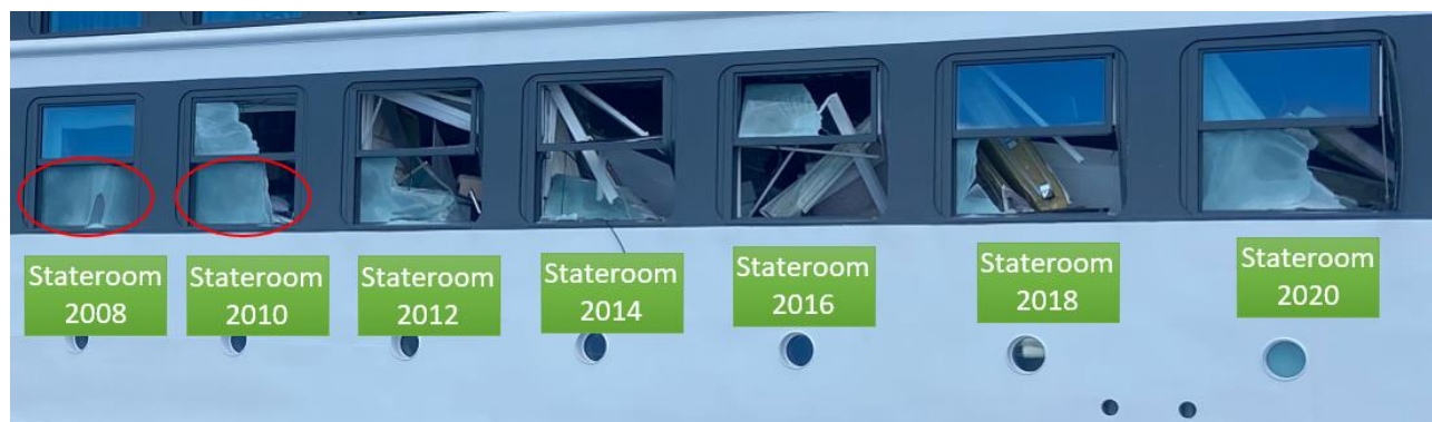
Figure 76: The windows where the window pane is broken but the frame is intact are circled in red. Photo: NSIA/consultant
