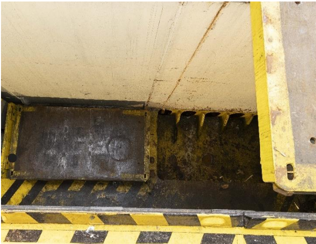
Figure 9: The lift shaft with the aft lift platform to the right of the photo, flush with the upper cargo deck. The forward lift platform parked on the lower cargo deck to the left of the photo. Photo: The police
