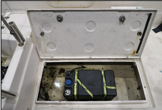
Figure 11: Flush hatch in the open position. Photo: NSIA
