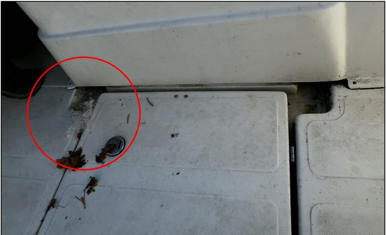
Figure 27: Image from the aft deck showing how the drainage channel around the main hatch merges with the aft drainage channels. The red circle shows water entering the deck through the starboard drain opening in sea conditions with a significant wave height of approximately 0.5 metres. Photo and illustration: NSIA
