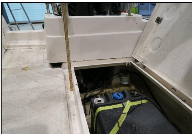
Figure 13: Drainage channels around the hatch coaming. Photo: NSIA
