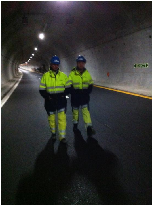
Figure 2: Tunnel incidents can have a great high injury potential. Photo from inspection of a new and modern tunnel on the E6. Photo: AIBN
