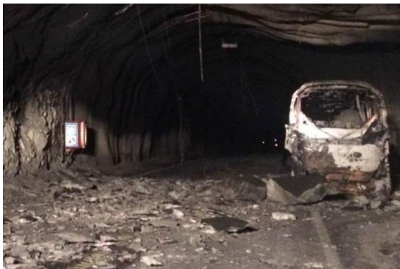
Figure 6: Fallen debris, viewed from the Flåm side. Photo: Aurland fire service
