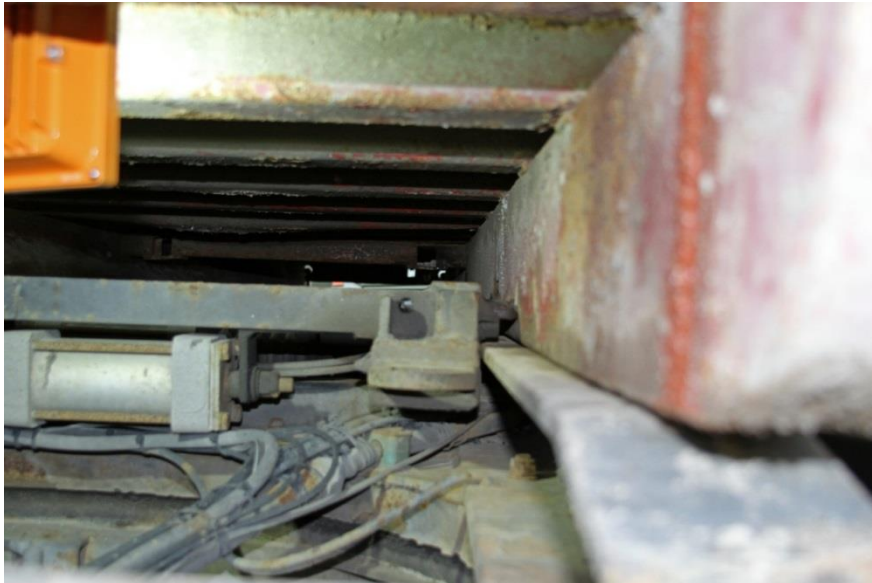
Photo 10. Trailer with hooklift container, observe that the front pair of securing devices do not have any holes to fit into in the container frame. The aft pair fits into holes in the frame of the container.
