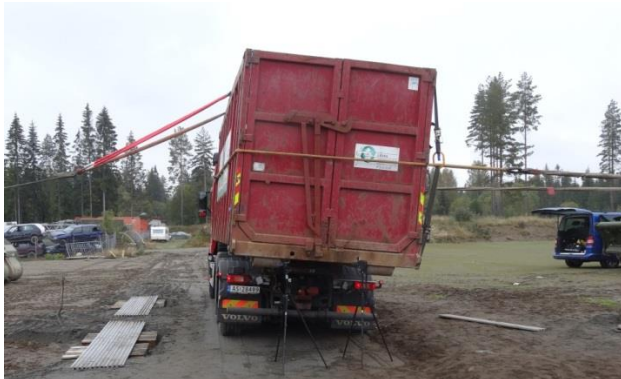
Photo 1. Truck with container. To the right of the container is the strap that is used to apply the lateral force. The other strap is only used to secure the vehicle from tipping.
