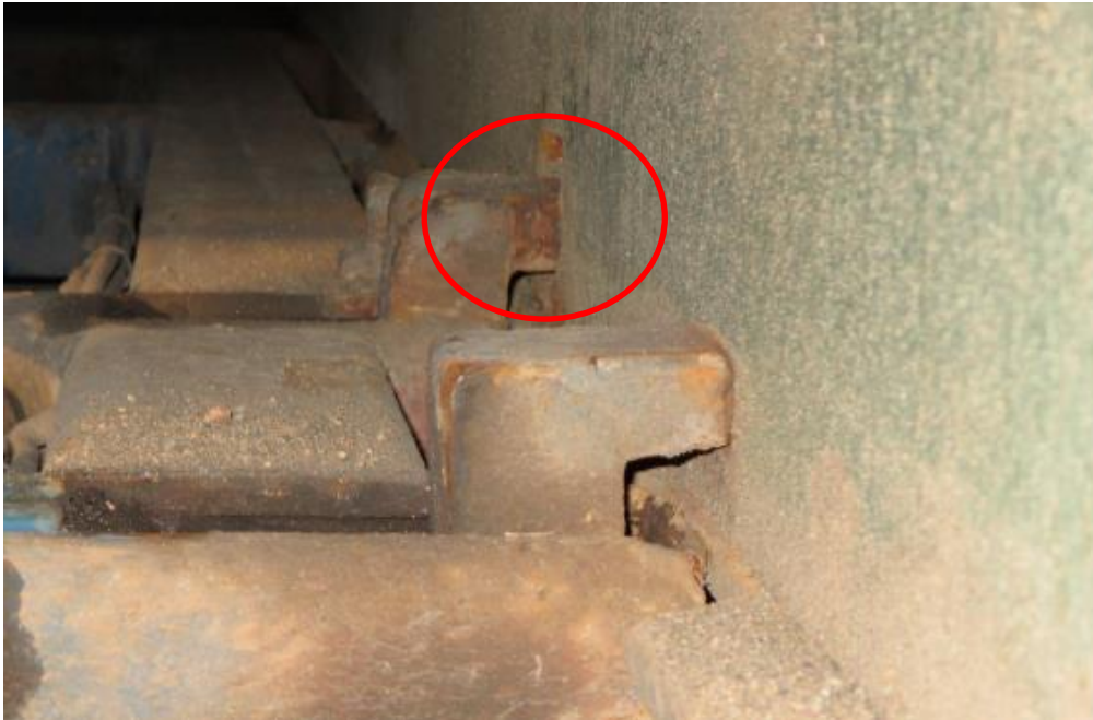
Figure 4: Marks on the locking stud from the container's lateral movements. Photo: NPRA Illustration: AIBN
