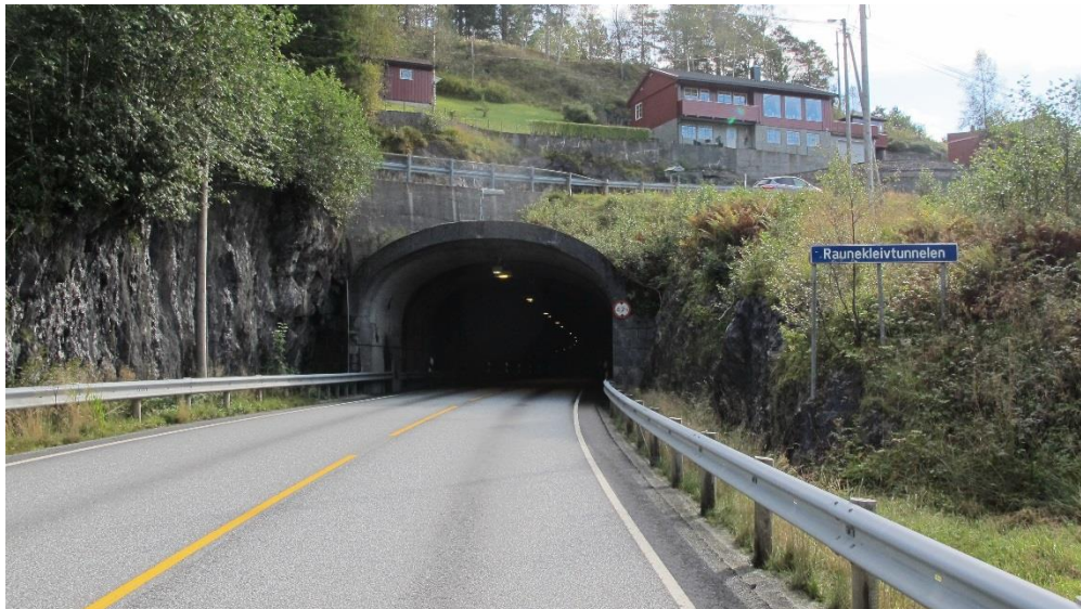
Figure 6: The photo was taken ten metres outside the tunnel opening. The light conditions when the photo was taken are very much like on the day of the accident. Photo: AIBN
