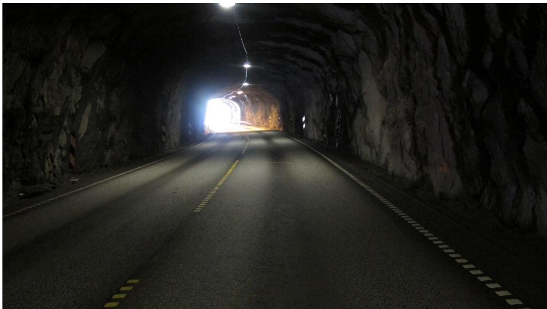
Figure 9: Road environment inside the Raunekleiv tunnel. Photo: AIBN
