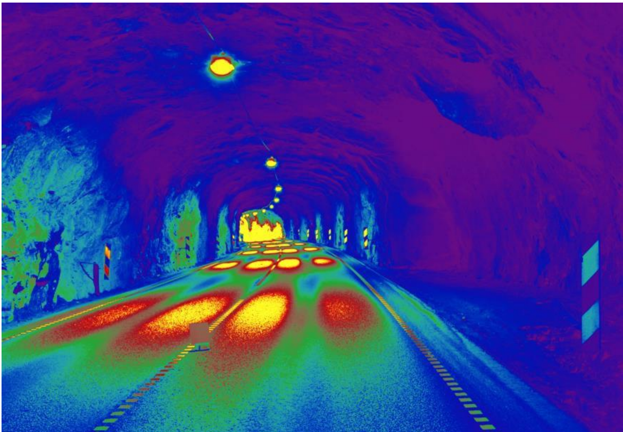
Figure 4. The image shows the transition zone in the Raunekleiv tunnel (approx. 100 metres from the tunnel portal) in false colours.
