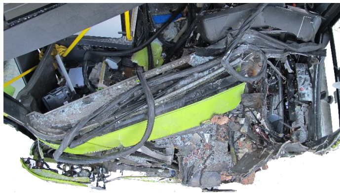
Figure 4: Deformations of the driver's cab in the eastbound bus, seen from above. Photo: AIBN
