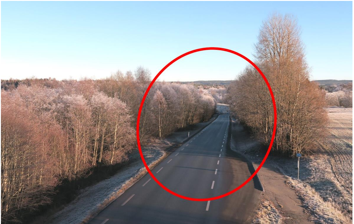
Figure 20: Area of shade seen facing east from Molstad bus stop down Nafstad hill towards the right-hand bend. The photo was taken at 12:30 on 26 November 2018 in subzero temperatures. Photo: AIBN
