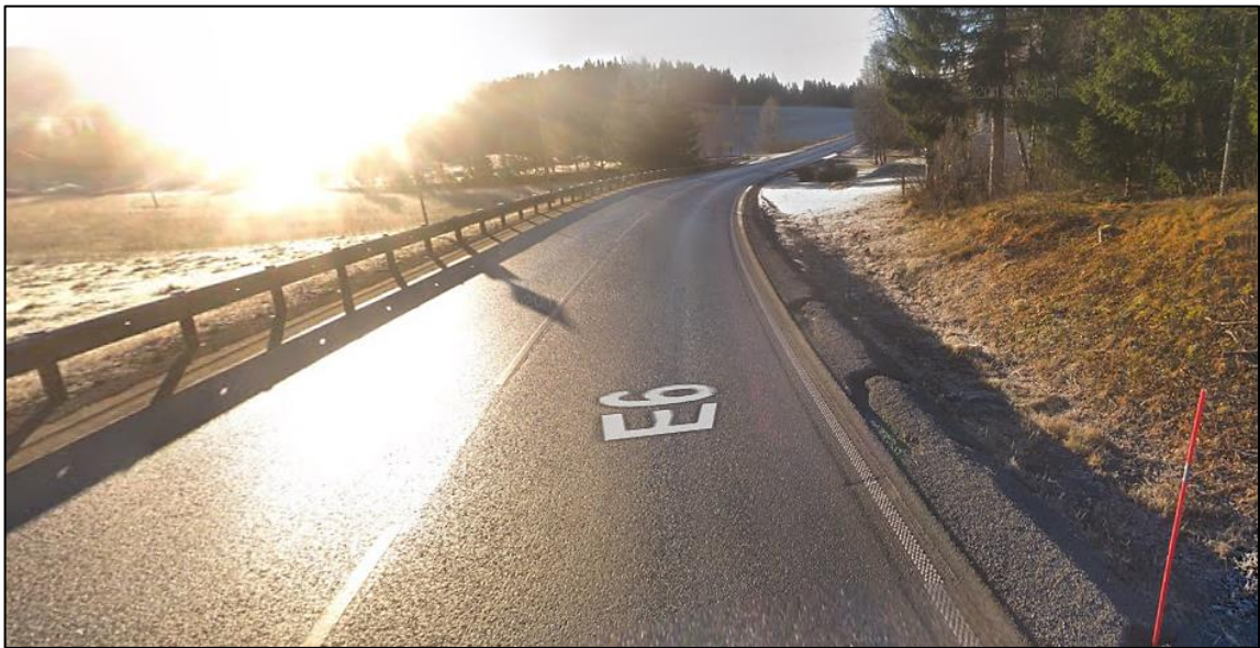
Figure 2: North-to-south view of the section of road where the heavy goods vehicles collided. Photo: Google Maps
