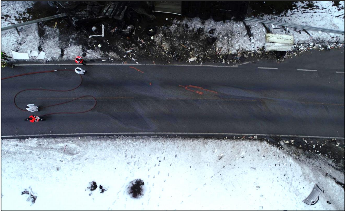
Figure 11: Marks left (indicated in orange) in the northbound lane. Photo: NPRA
