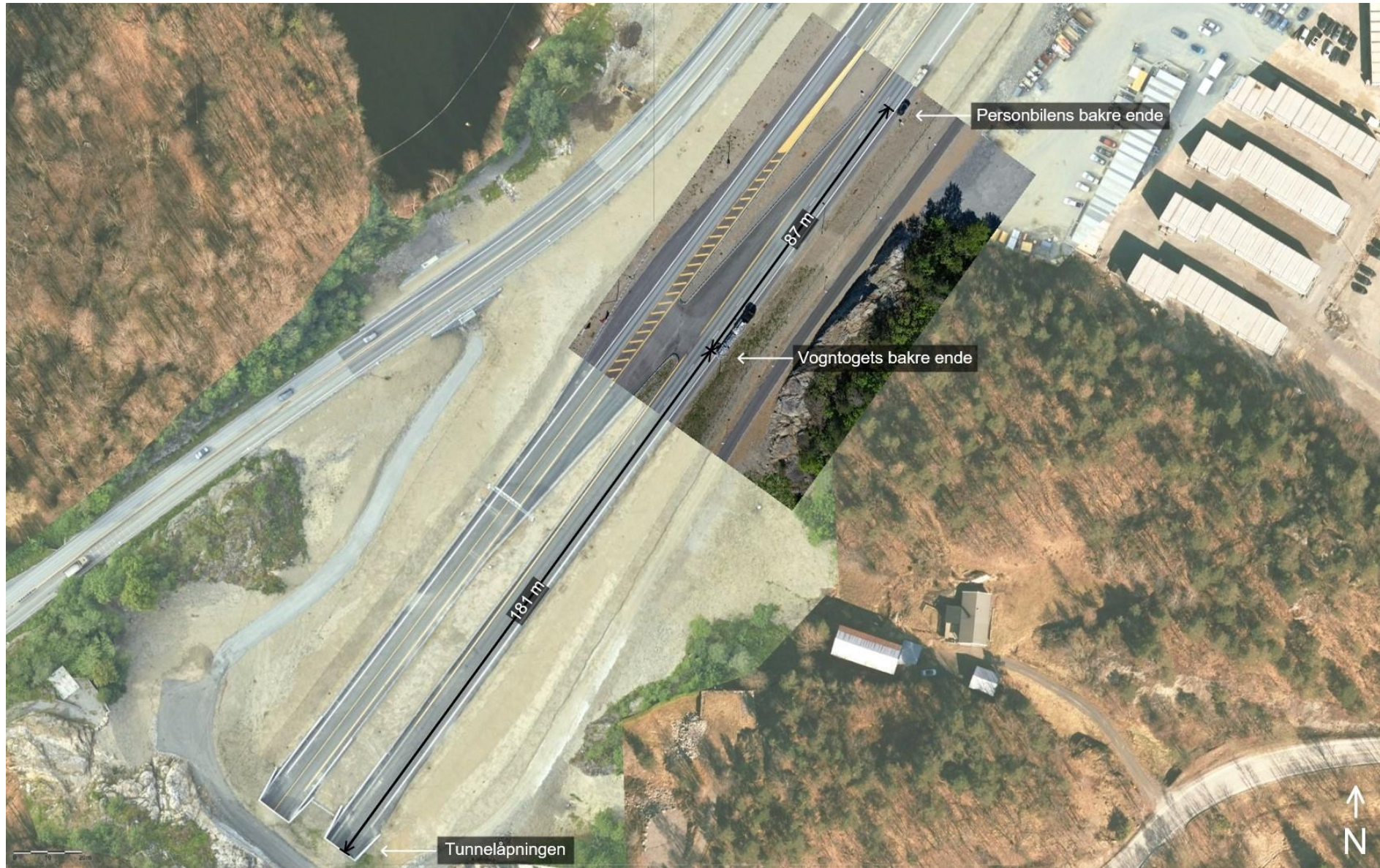
Figure 8: Overview photo and drone photo of the accident site. Map: © Norwegian Mapping Authority. Photo: The police. Illustration: NSIA
