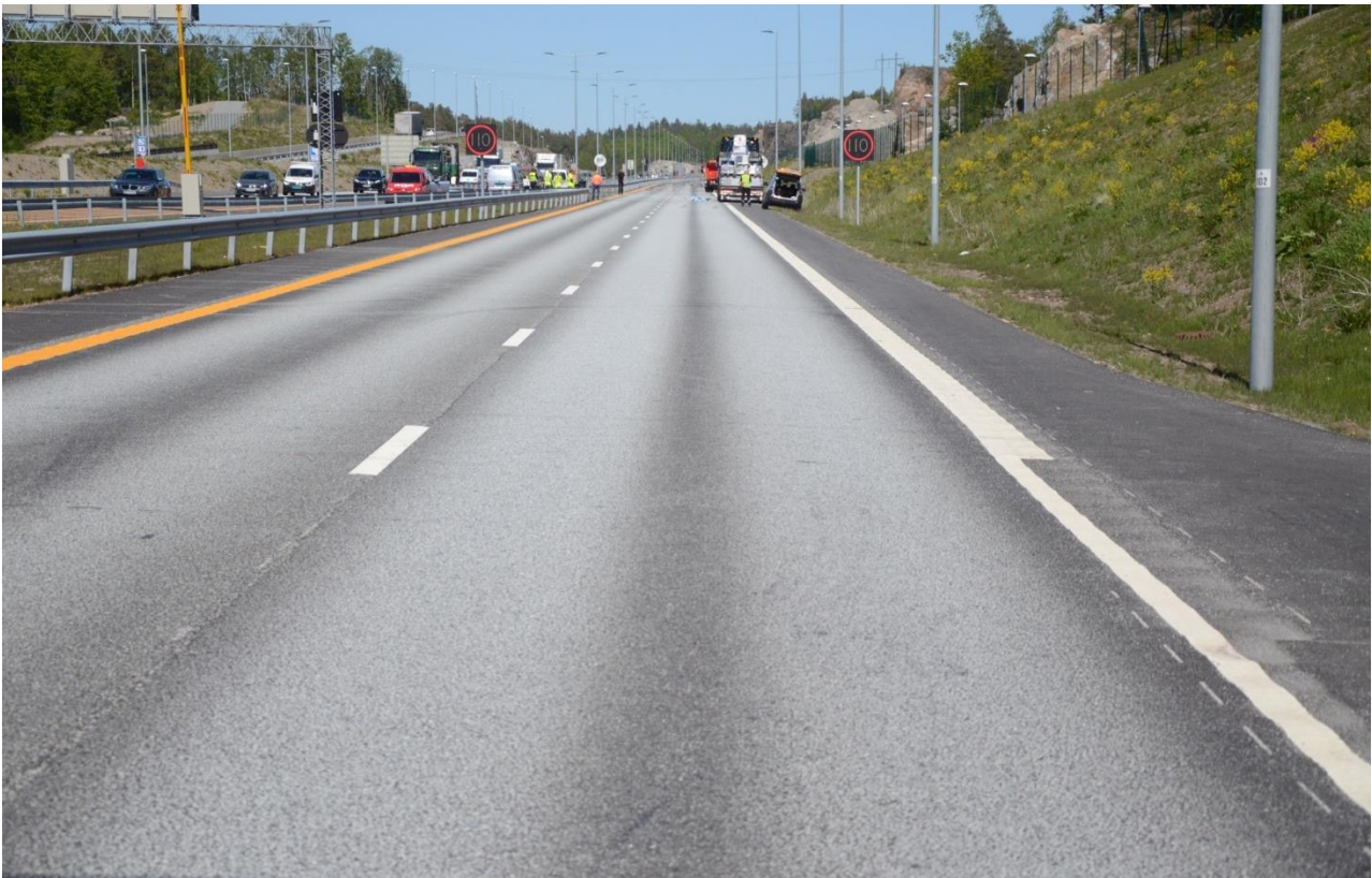
Figure 23: Visibility from the tunnel portal, 181 metres from the HGV. Photo: The police
