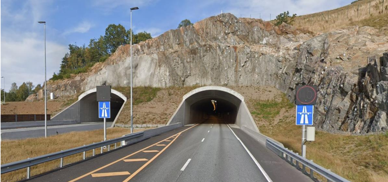
Figure 19: The portal of the Torsbuås tunnel with electronic speed limit signs, view when travelling north. Photo: Google Maps
