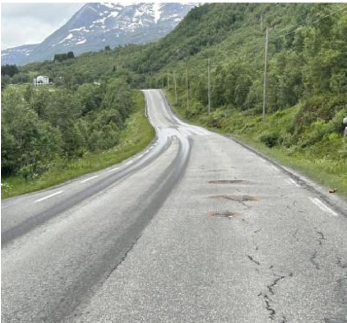
Figure 5: The accident site on the E10 in Tjeldsund with bumps in the road surface and rocks in the roadside terrain. Photo: The police
