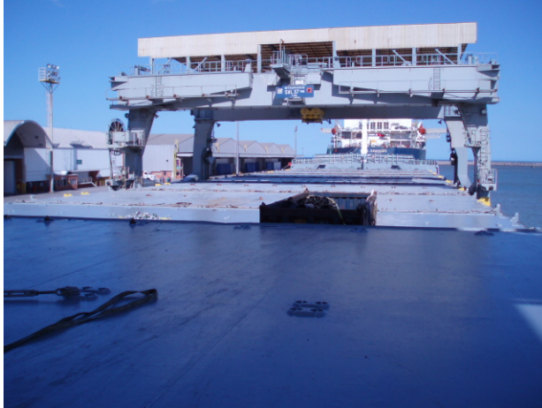
Figure 5: Partially enclosed gantry crane.
