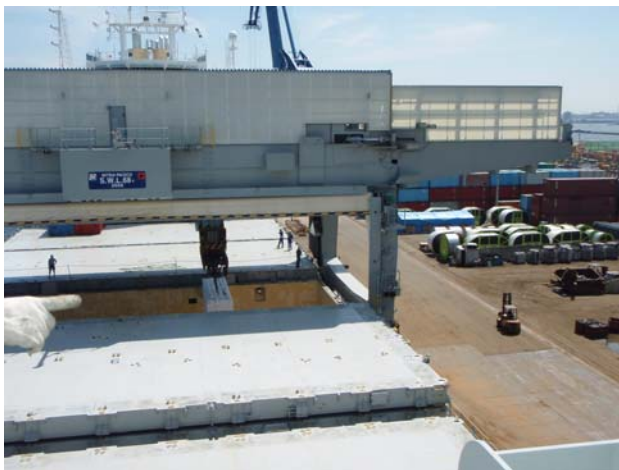
Figure 6: Enclosed gantry crane.
